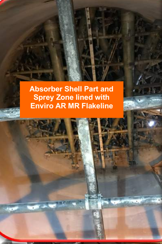
%98 Sulfuric Acid Absorber lined with Enviro AR MR Flakeline
